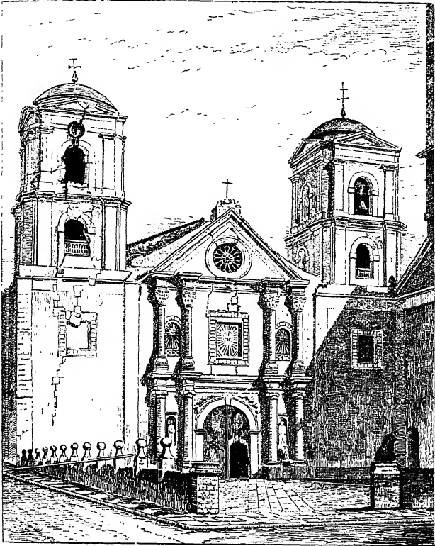
FIG. 22.—Church of St. Augustin, Manilla. Earthquakes of July 18-20, 1880.
